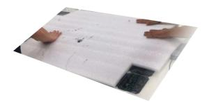
Apply adhesive around the panel after installation.
